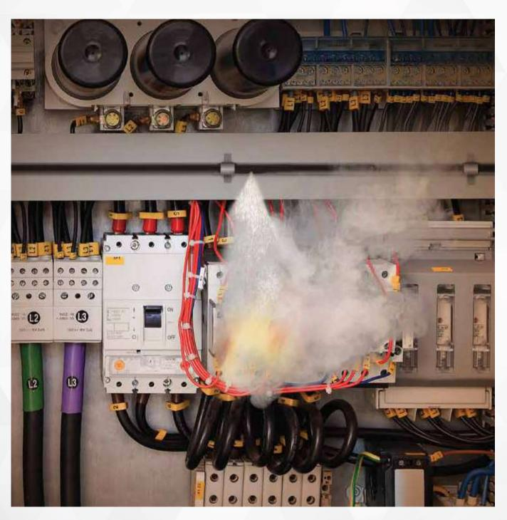
IN-PANEL TUBE BASED MICRO-ENVIRONMENT SUPPRESSION SYSTEM (CQRS)
