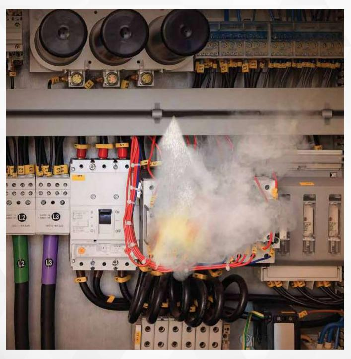
IN-PANEL TUBE BASED MICRO-ENVIRONMENT SUPPRESSION SYSTEM (CQRS)
